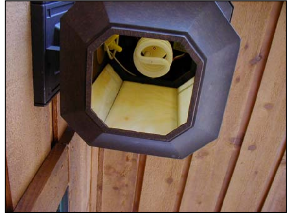
Code compliant—bulb is shielded and downcast
