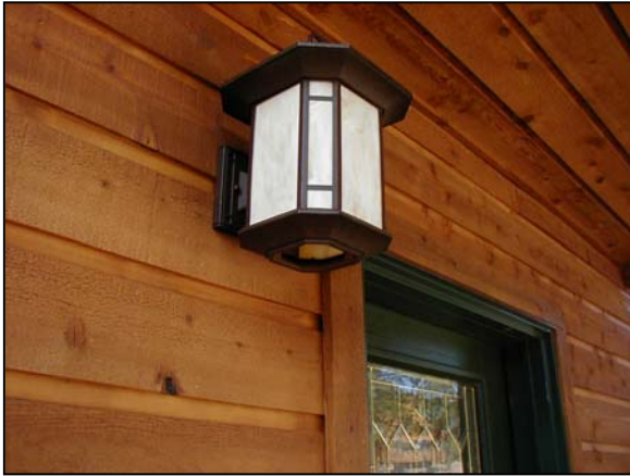
Code compliant—bulb is shielded and downcast
