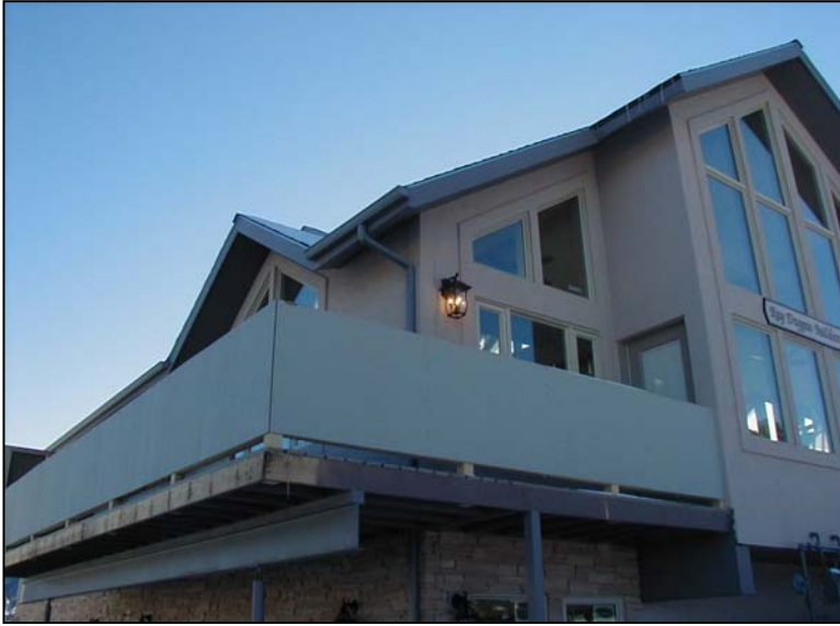
Not code compliant—bulb is visible
