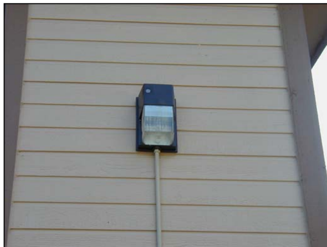
Not code compliant—bulb is not cut off and optics are designed to reflect light outward
