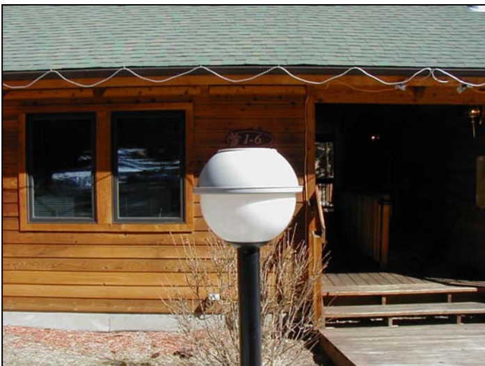
Code compliant—bulb is shielded and downcast
