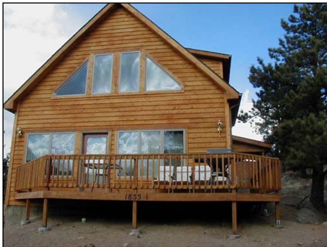
Code compliant—bulb is shielded and downcast
