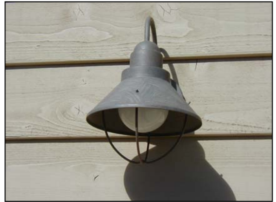
Code compliant—bulb is shielded and downcast
